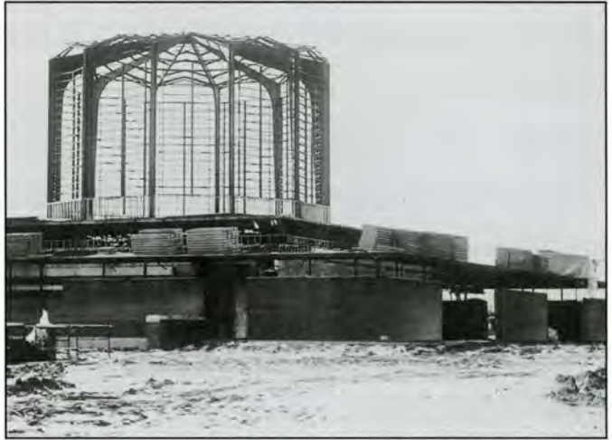
Elmwood Avenue Temple under construction, 1961. (Courtesy Rochester Public Library)
